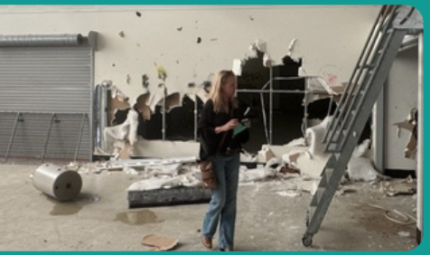
Inspecting the TAFE interiors following reassessment
